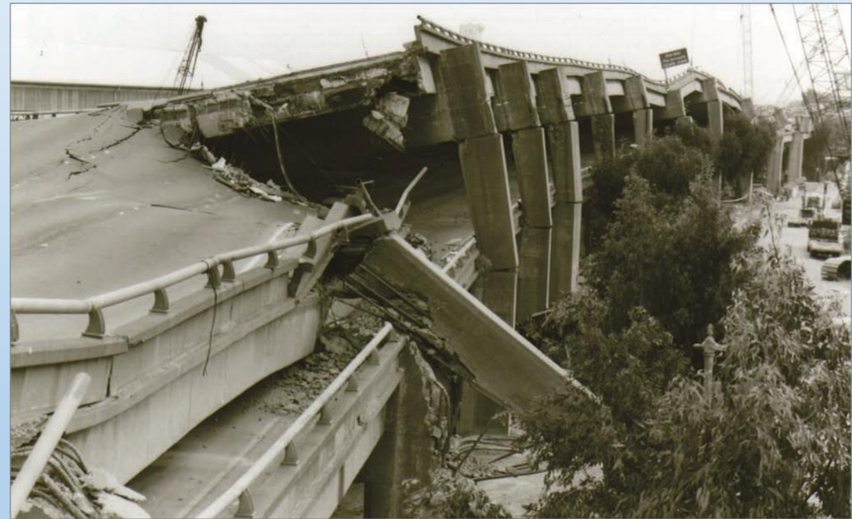
FIGURE 7: Collapsed Section of the Cypress Street Viaduct
