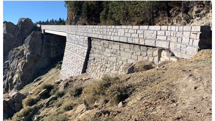
FIGURE 18: Completed Echo Summit Bridge
