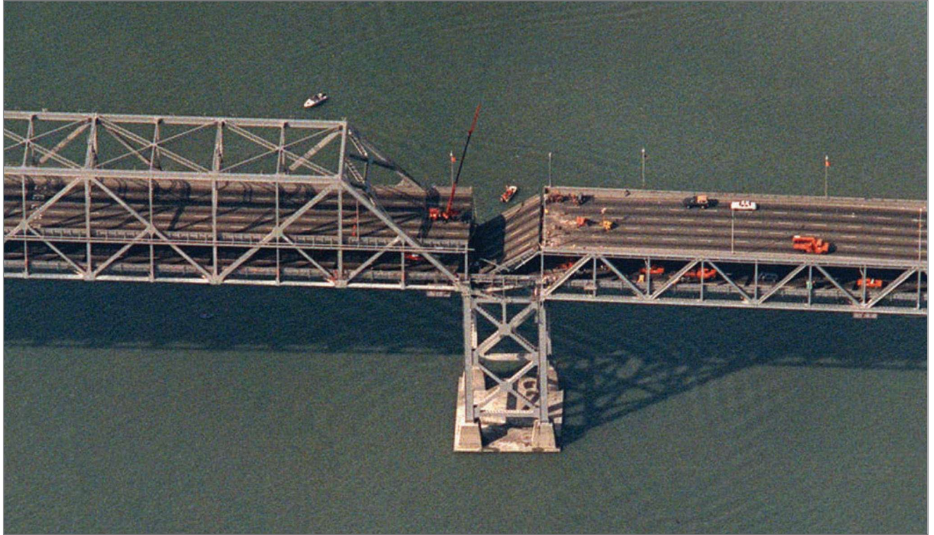
FIGURE 8: San Francisco–Oakland Bay Bridge Insufficient Hinge Seat
