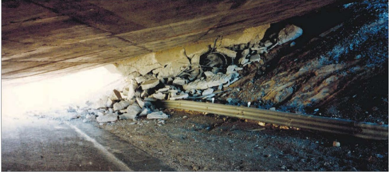
FIGURE 10: Failure of a Short Column at the I-14/I-5 Connector Separation and Overhead
