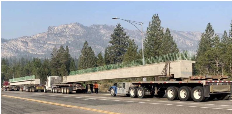
FIGURE 17: Echo Summit Precast Girders
