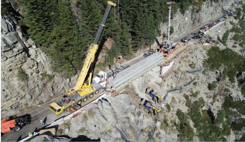
FIGURE 16: Echo Summit Bridge Replacement Project
