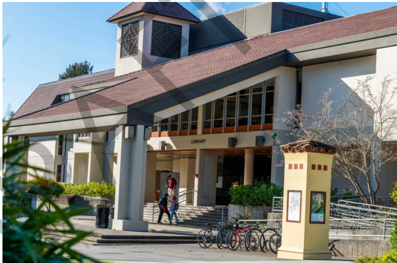
Figure 5 Cal Poly Humboldt Library Renovation
