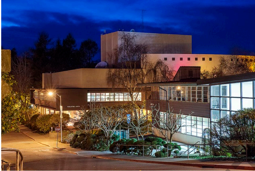
Figure 6 Cal Poly Humboldt Theater Arts renovation
