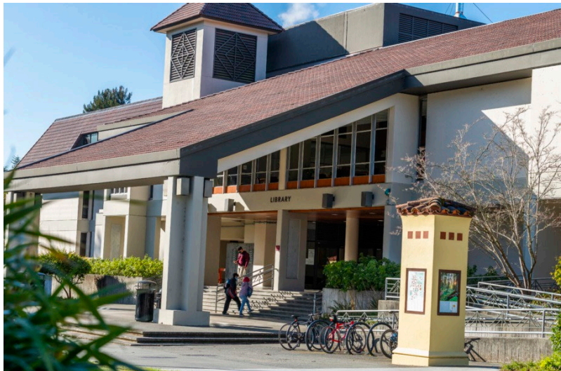
Figure 5 Cal Poly Humboldt Library Renovation
