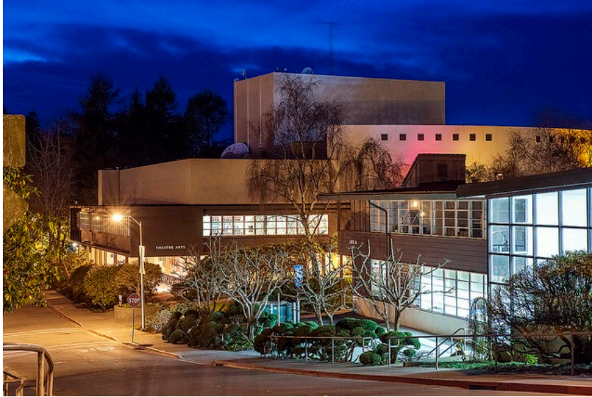
Figure 6 Cal Poly Humboldt Theater Arts renovation
