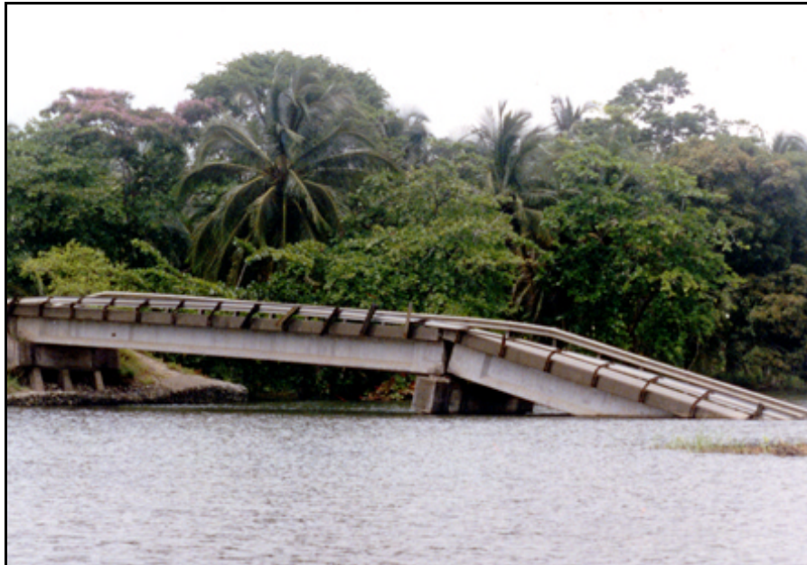
Figure C-7: Bridge Destroyed by Lateral Spreading, 1991 Limón, Costa Rica earthquake (courtesy EQE International, Inc.)
