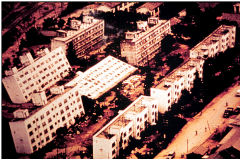
Figure C-6: Apartment buildings damaged by liquefaction, 1964 Nigaata earthquake (courtesy EQUIIS Photographic Database)
