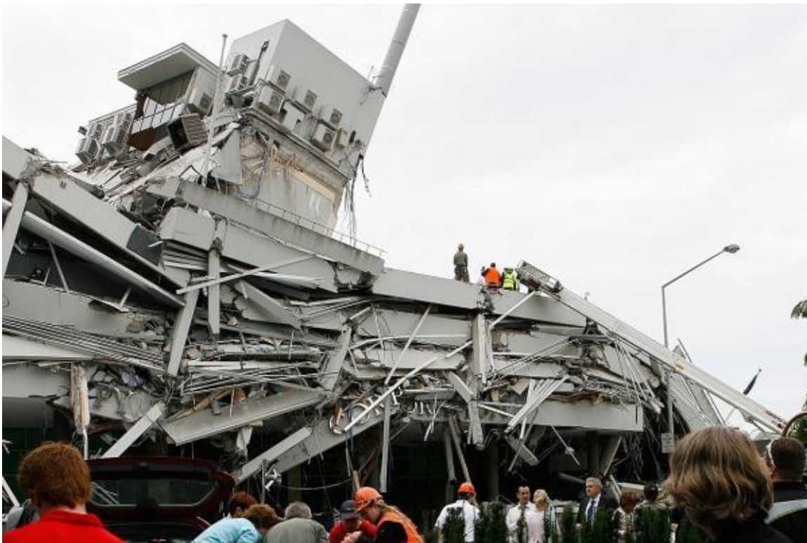
The collapse of the Pyne Gould Building in Christchurch, New Zealand in 2011 killed 18 people. It was a non-ductile concrete building that had been partially retrofitted before the earthquake.
