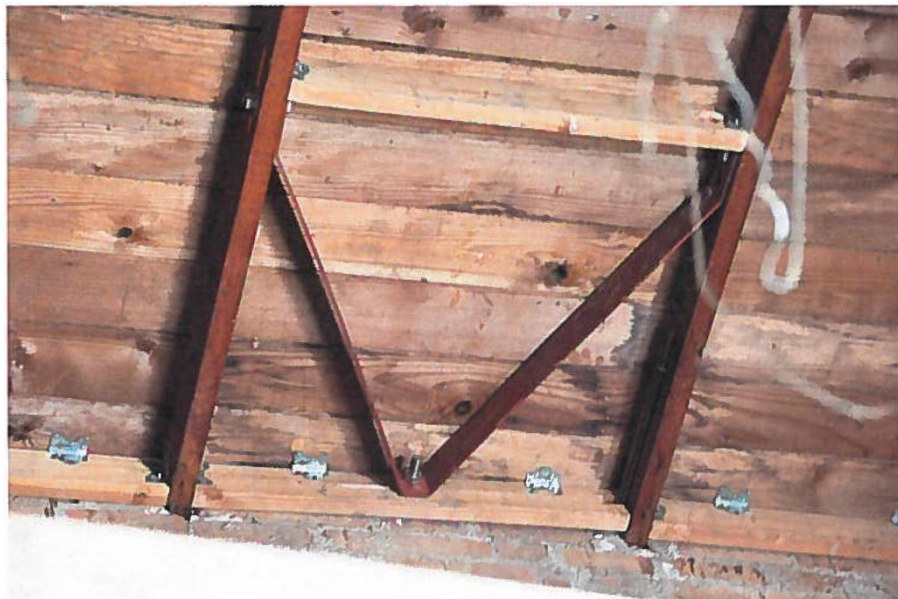
Retrofits often include adding new connections of walls to roofs.
