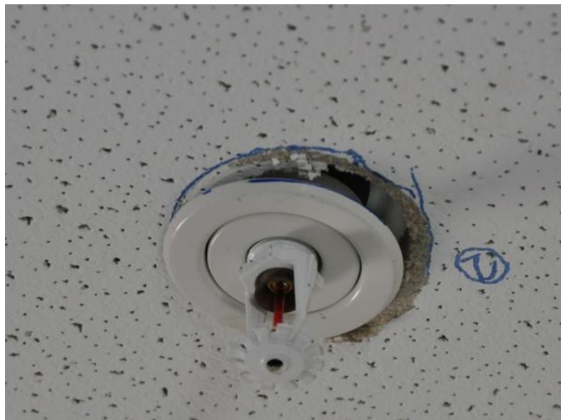
Ceilings that move during earthquakes can shear off sprinkler heads, causing water damage.
