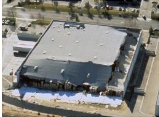
Precast (tilt-up) buildings, built primarily before 1995, may have reinforced concrete walls that are poorly anchored to roofs.
