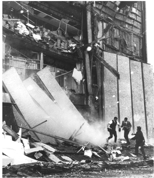
Failure of improperly attached cladding.
