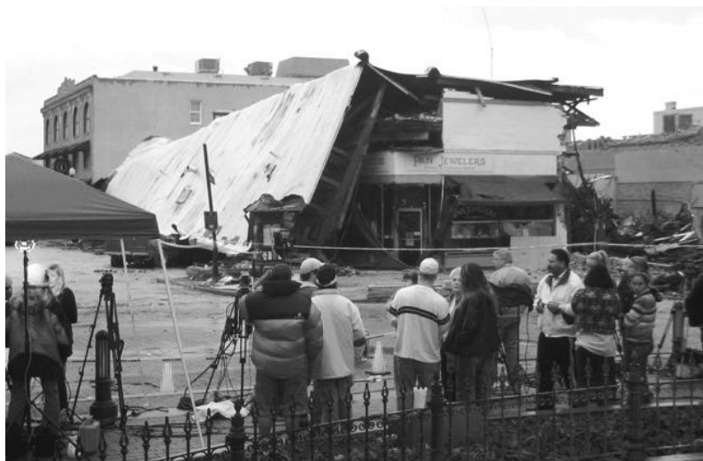
Collapse of the Acorn Tower Building, Paso Robles, after the 2003 San Simeon earthquake.
