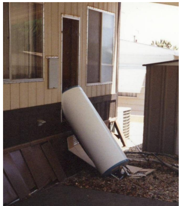
Failure of unbraced water heater.
