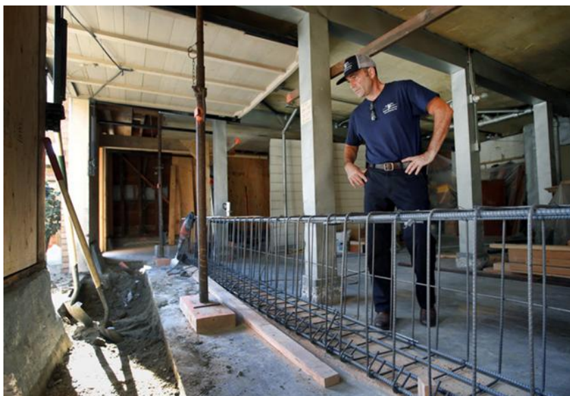
Soft story apartment building with a retrofit underway.
