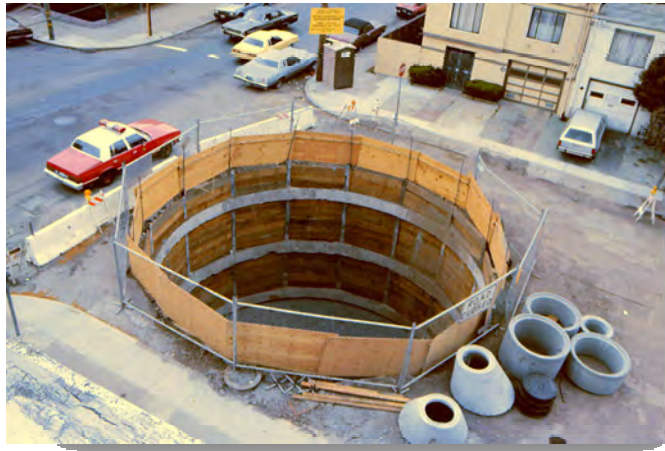
Figure 36 Typical San Francisco Fire Department cistern under construction.
