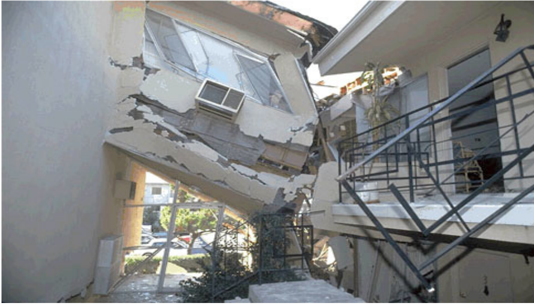
Apartment building damaged during Northridge earthquake.
