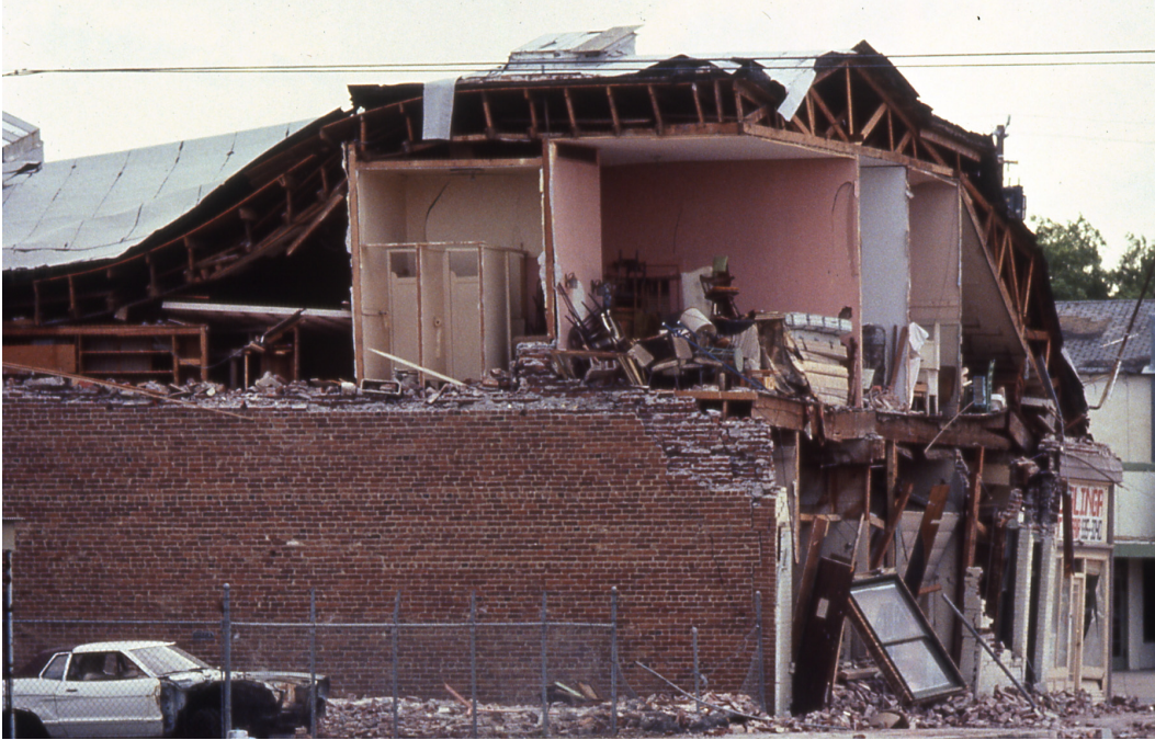
Heavy wall construction collapse.
