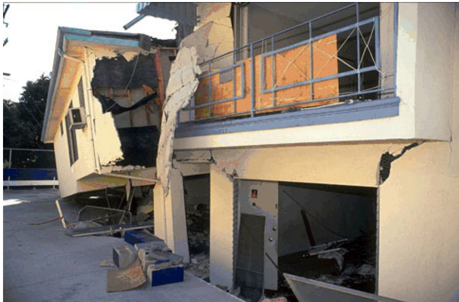
Light frame construction collapse.
