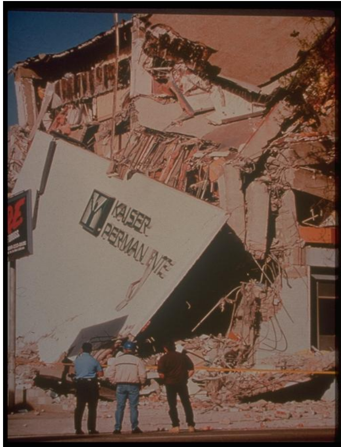
Heavy floor construction collapse.
