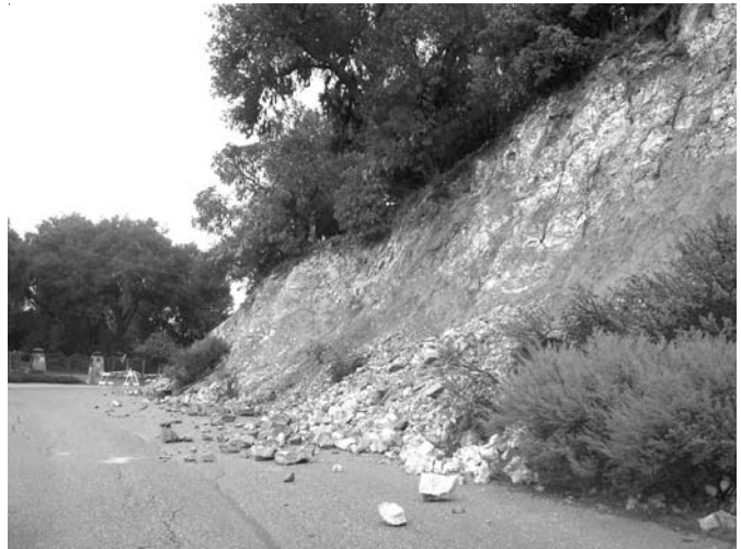
Figure 65 - Landslide. San Simeon Earthquake, December 22, 2003 Landslides on San Gregorio Road in Atascadero, California, only a short distance away from where the commercial properties with the most damage were located.
