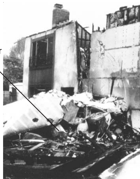
Figure 10 - The unbraced water heater in this building fell during an earthquake; the resulting fire destroyed the building.
