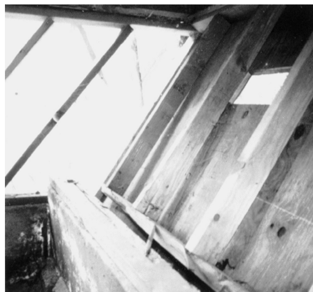
Figure 23 - This photograph shows an interior detail of a home similar to the one above, showing substantial damage to a building with an unbraced tall wall.
