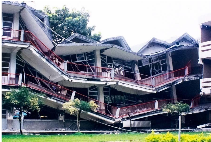
Figure 3: Damage to High School during the 1999 Chi-Chi Earthquake. (This collapsed school building has now been converted into a national museum.) (Photo Credit: Wei-sen Lee, National Science and Technology Center for Disaster Reduction, Taipei, Taiwan)
