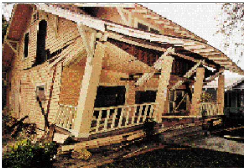
Figure 44. Older homes with horizontal wood siding are particularly vulnerable to damage if they are not securely fastened to a proper foundation.
