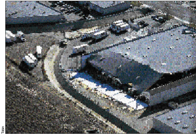
Figure 22. This industrial tilt-up building had its roof and wall partially collapse.
