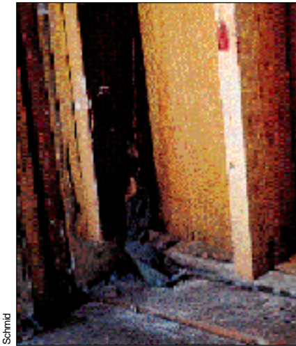
Figure 51. This metal connector stretched, distorted, and eventually caused the wood to split.
