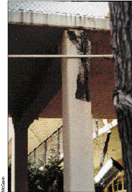
Figure 61. Damage to a concrete column on a two-story elevated walkway at Patrick Henry Junior High School. Note the failure of the guardrail in the background.
