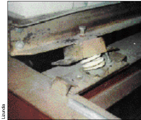
Figure 28. Broken supports on heating and ventilating equipment can render this equipment useless.
