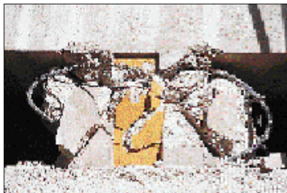
Figure 55. Short columns in this parking structure failed. Modern building codes now require much more reinforcing steel for such short columns.
