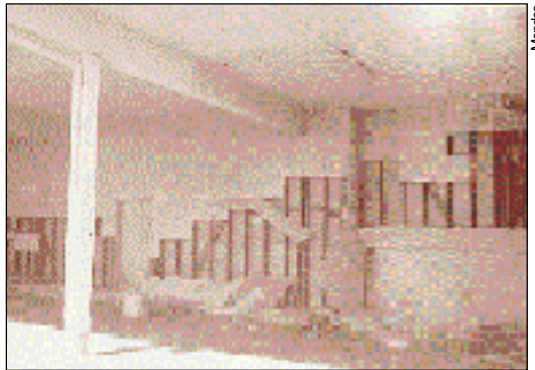
Figure 42. Walls in this building were repaired and retrofitted with plywood after 1971. In 1994 it suffered only minor damage.
