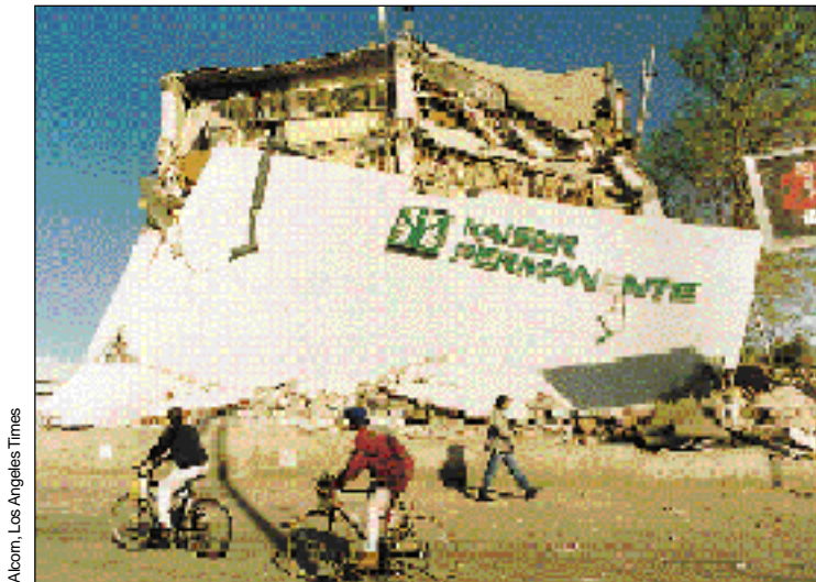
Figure 33. Both ends of this 1960s medical office building collapsed and the second floor “pan-caked.” Fortunately it was not occupied.
