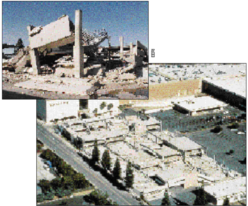
Figure 16. This shopping mall parking structure collapsed primarily because its parts were not connected to each other. Inset , close-up of the same parking structure, showing separation of components.
