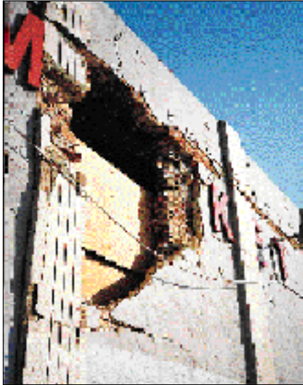
Figure 35. Although this retrofitted building lost a few bricks and may be difficult to repair, damage was significantly less than in similar unreinforced buildings. The outer layer of brick was not adequately connected to the inner layers.
