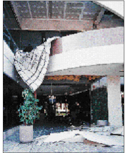
Figure 26. Heavy plaster ceilings or soffits can pose serious risks to occupants.
