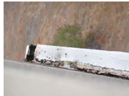
Fig. 2(c) Gap between exterior CFS framed wall system created due to ground motion and soot from smoke
