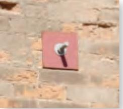
A steel plate with anchor bolts.
