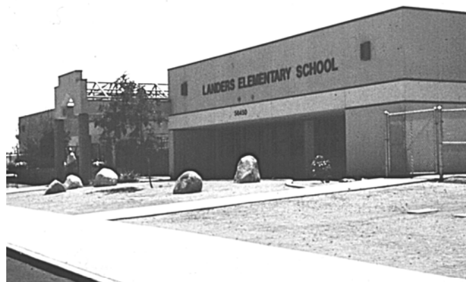
Figure 4 Landers Elementary School with minor non-structural damage and immediate reuse after the 7.3 magnitude 1992 Landers earthquake. There has been no partial or full collapse of any public school building constructed to the requirements of the Field Act since 1933.
