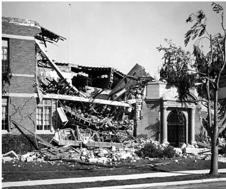
Figure 1 Jefferson Junior High School damage after the 6.4 magnitude 1933 Long Beach earthquake.
