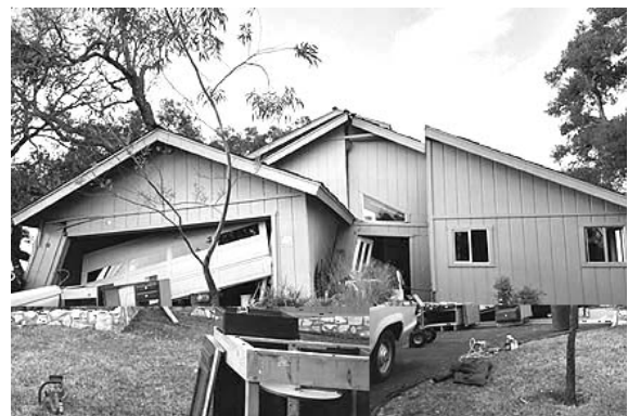
Figure 5 - San Simeon Earthquake, Dec. 22, 2003 This home slid two feet off its foundation due to inadequate nailing of walls to its sill plates.
