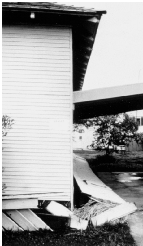
Figure 15 - Damage to home due to cripple wall failure.
