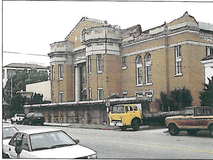
Figure 76. The historic First Christian Church in Santa Monica was seriously damaged in the earthquake.
