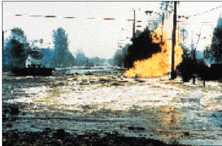
Figure 71. Fire and flood produced calamity at Balboa Boulevard's ruptured gas and water mains.
