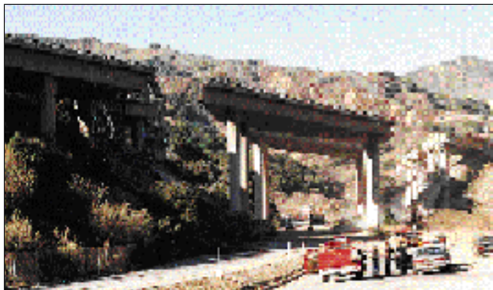
Figure 70. Deck sections fell off their seats at the Gavin Canyon Undercrossing on I-5.
