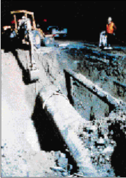
Figure 73. This four-foot-diameter water main under Balboa Boulevard buckled and ruptured when surrounding soils compressed it.
