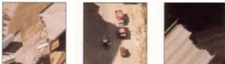
% Roadbed sections of part of Interstate 5 fell off their supports.
