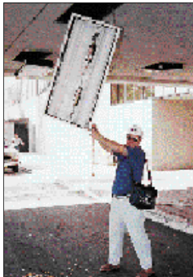
Figure 32. A light fixture partially fell when an anchor for one of its two safety wires pulled out at the Sylmar County (Olive View) Hospital.
