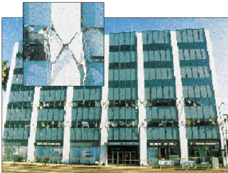
Figure 53. This office building's exterior cladding affected the way its frame responded to shaking, finally resulting in column failure and demolition. Inset , detail.
