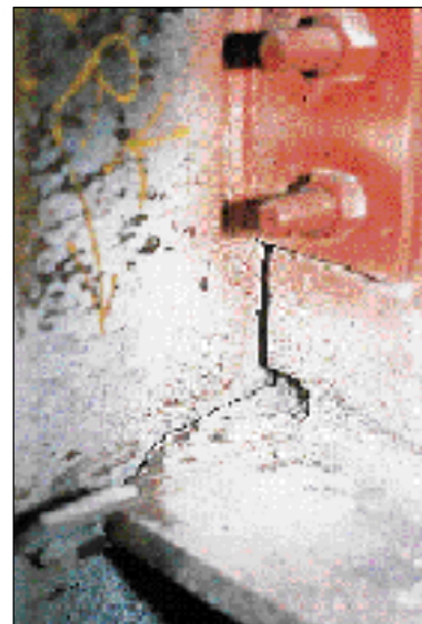
Figure 56. Steel-frame connections were unexpectedly cracked.
