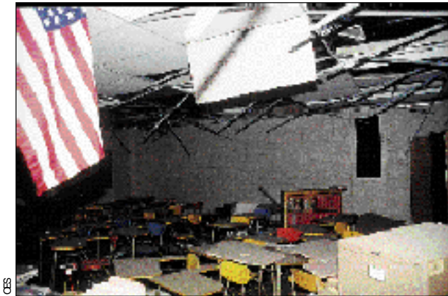
Figure 25. Though falling acoustic ceiling tiles like this are not particularly dangerous, falling light fixtures and other heavier elements can be.
