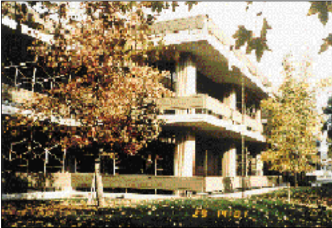
Figure 40. This building in Santa Clarita is shown during its 1993 retrofit which was undertaken with minimal disruption to its occupants. The building emerged from the Northridge earthquake with no structural damage.
