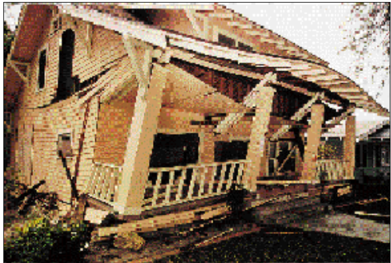
Figure 44. Older homes with horizontal wood siding are particularly vulnerable to damage if they are not securely fastened to a proper foundation.
