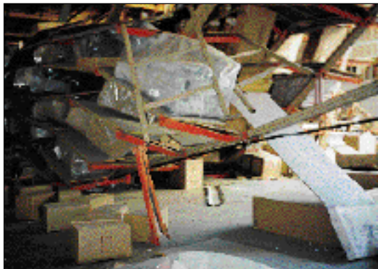
Figure 29. Collapsed storage racks would have posed substantial risks to life had this building been occupied during the earthquake.
