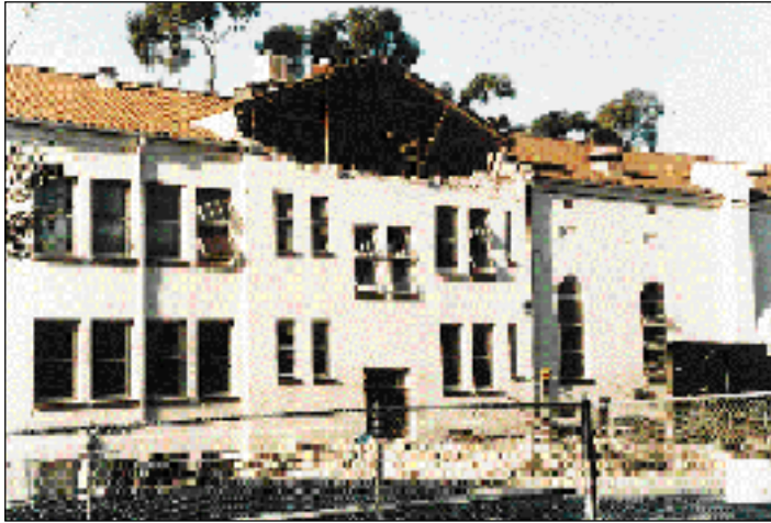
Figure 66. Life-threatening structural hazards such as this are still allowed in older private schools throughout California. Most of them have been eliminated in our public schools.
