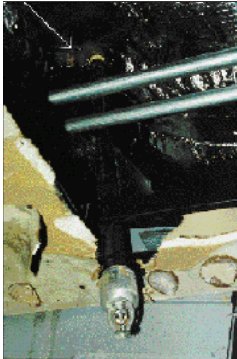
Figure 59. Water from failed sprinkler lines produced costly damage and disruption.
