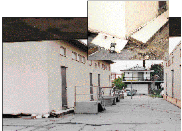
Figure 62. Several portable classrooms were seriously damaged after falling from weak or poorly maintained foundations. Inset, detail.
