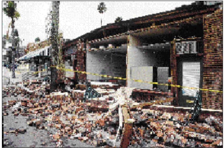
Figure 36. The entire facade of this unretrofitted brick building in Fillmore was lost. The city contemplated requiring retrofit measures but concluded as recently as 1993 that they were economically prohibitive.
