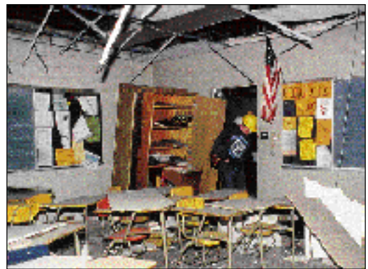
Figure 65. Though less life-threatening than light fixtures, ceiling tiles were a major property loss that could have been reduced with modern bracing techniques.
