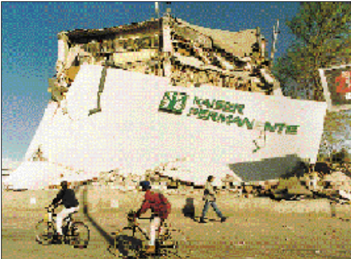
Figure 33. Both ends of this 1960s medical office building collapsed and the second floor “pan-caked.” Fortunately it was not occupied.
