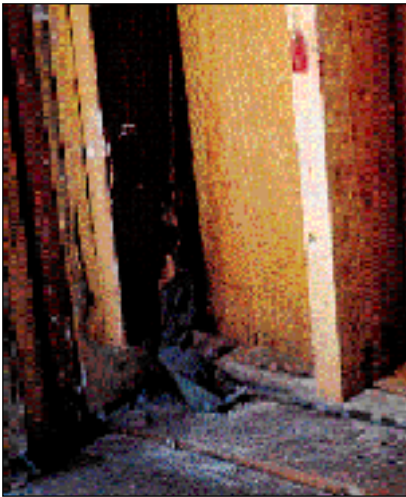
Figure 51. This metal connector stretched, distorted, and eventually caused the wood to split.
