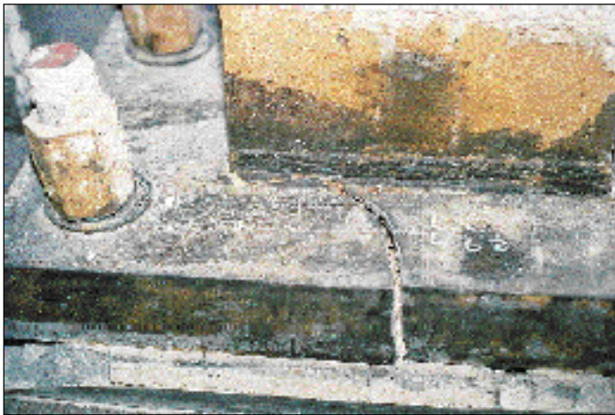
Figure 15. A 4-inch-thick steel plate supporting the base of a column at the Oviatt Library at CSU Northridge. The plate fractured when the building was violently shaken.
