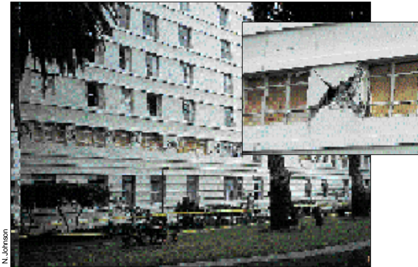
Figure 58. This older hospital was severely damaged. Lightly reinforced concrete walls lost much of their strength when X cracks formed. Inset, detail.
