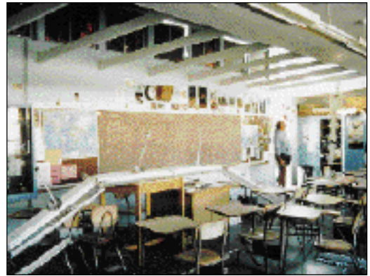
Figure 64. Falling light fixtures in over 100 classrooms would have posed significant threats to students and teachers had the earthquake occurred during school hours.
