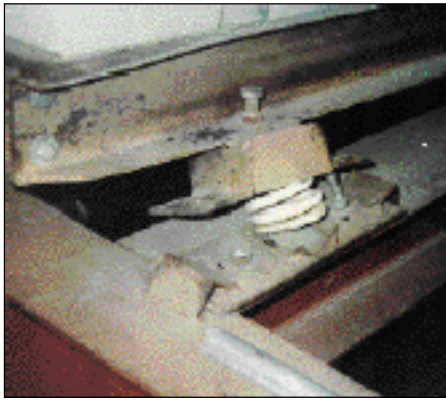
Figure 28. Broken supports on heating and ventilating equipment can render this equipment useless.
