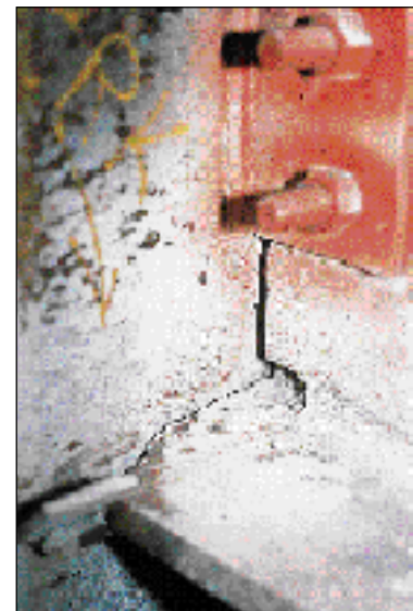
Figure 56. Steel-frame connections were unexpectedly cracked.
