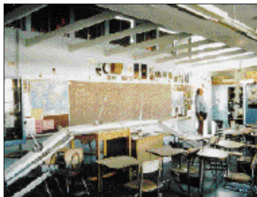
Figure 64. Falling light fixtures in over 100 classrooms would have posed significant threats to students and teachers had the earthquake occurred during school hours.
