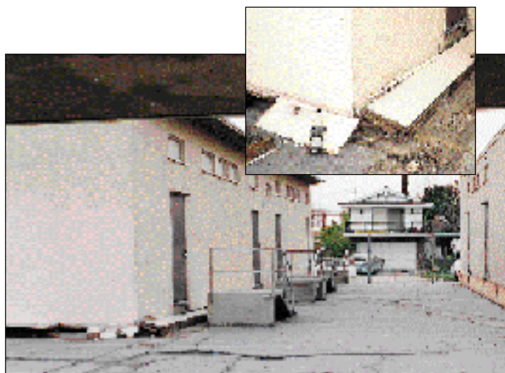
Figure 62. Several portable classrooms were seriously damaged after falling from weak or poorly maintained foundations. Inset, detail.
