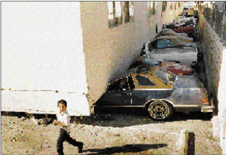
Figure 45. Older apartments like this with tuck-under parking collapsed because they were poorly braced.
