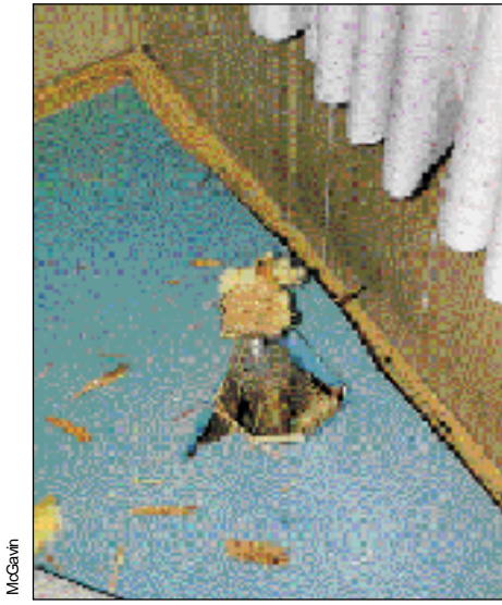
Figure 48. A steel jackstand pokes up through the floor of a mobile home after it shifted.
