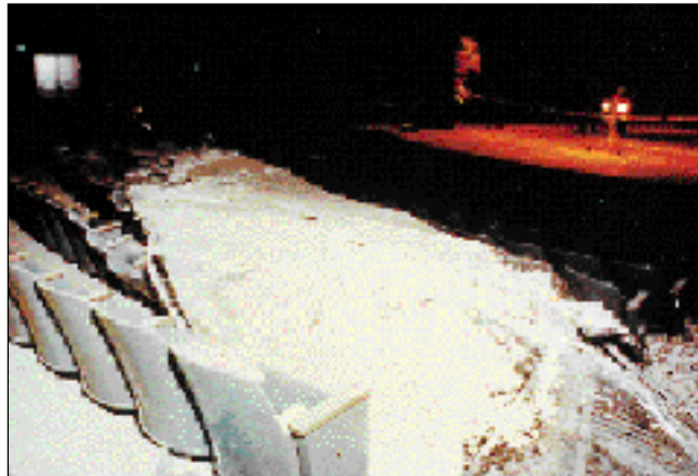
Figure 67. Large sections of a heavy plaster ceiling came down in Royce Hall. At another time of day, injuries and possibly deaths would have resulted.
