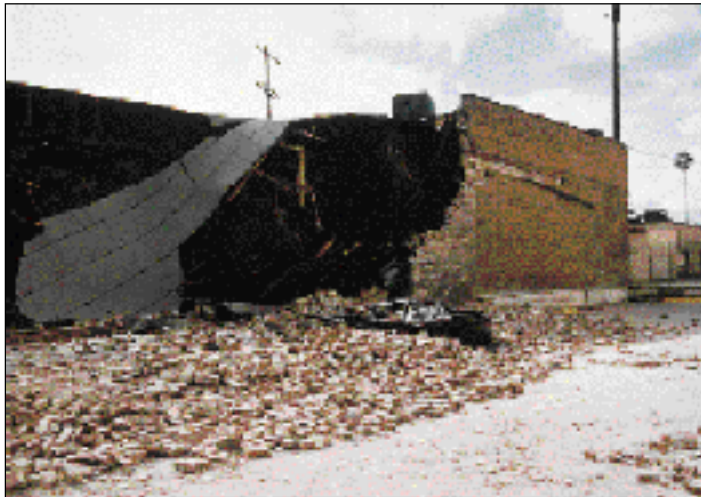
Figure 37. This retrofitted brick building collapsed in part because its wall braces were ineffective.
