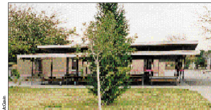
Figure 63. The lunch shelter at Danube Elementary School leaned over about one foot.
